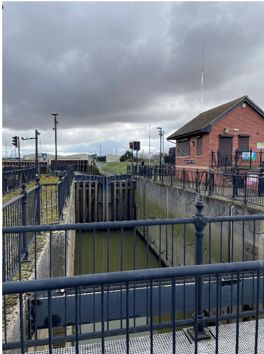
(Photograph 13 – Sluice gate, also used as a navigational lock, at Black Sluice Complex; facing east)
