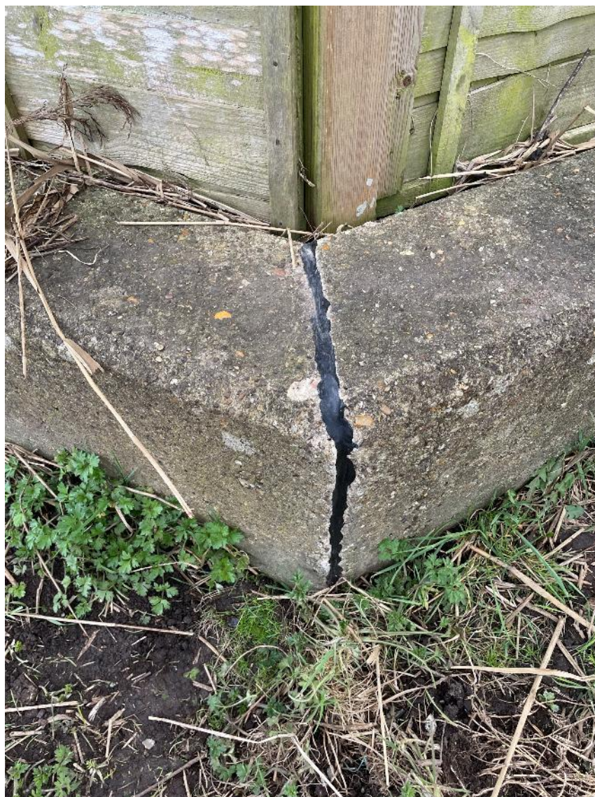
(Photograph 4 – Replaced seal on the eastern section of flood wall along the SFFD)
